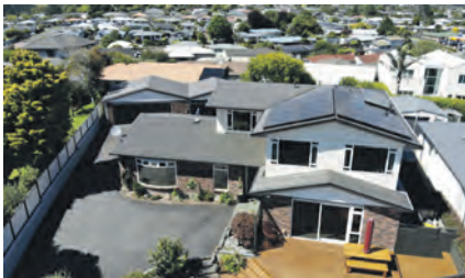
LEFT: A solar installation in a Coastal urban dwelling.
