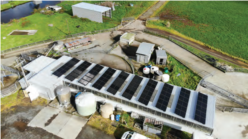
A completed solar installation on a dairy farm roof. Another first class effort by Sinclair Electrical.
